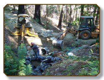
Temporary stream diversion for culvert installation
