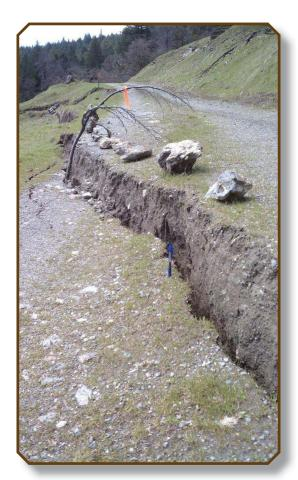
Poor road drainage led to slippage
